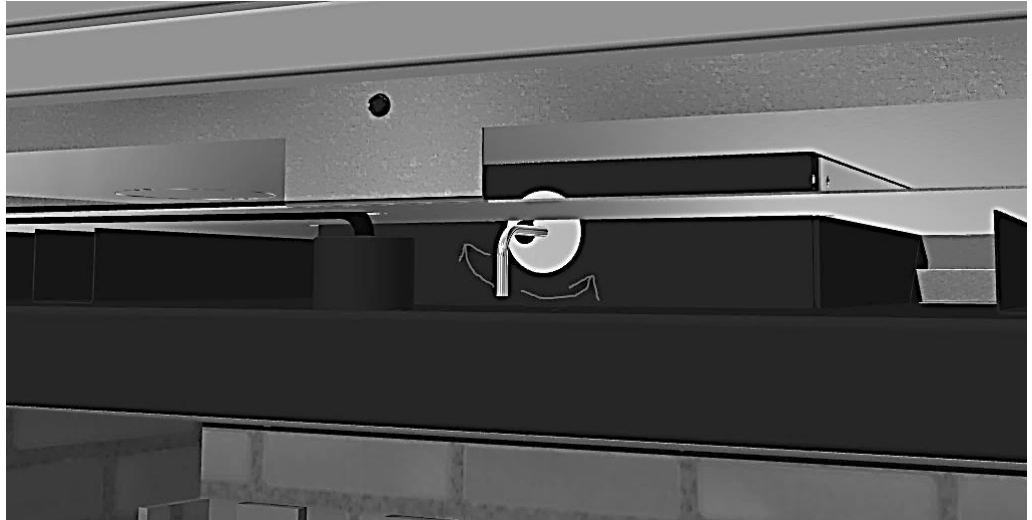
Figure 4-14 Exhaust Damper Adjustment
